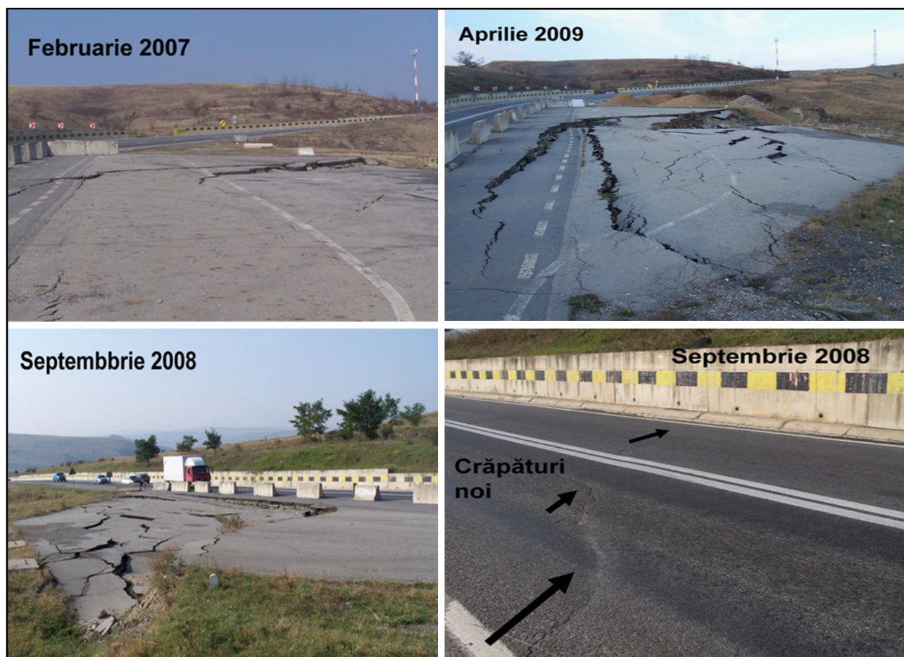
Fig. 126. Recent landslide (2005-2006) affecting the European road E81
