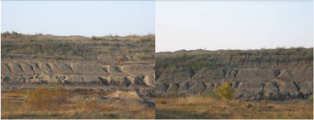
Fig. 26. Gully erosion on the Băișoara tailing dam embankment
