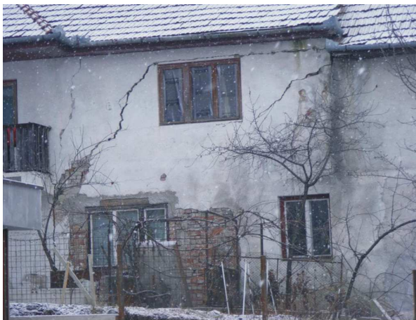
Fig. 8. Cracked house (Rosetti street, 2008)
