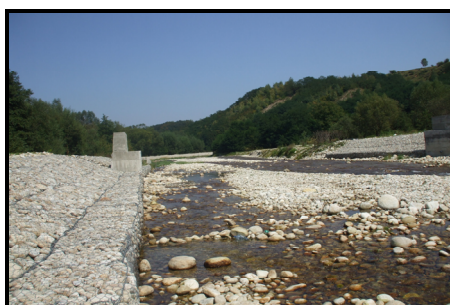
Photo 4. Embankment works of the Sibisel, upstream Sampetru (Santamarie-Orlea commune)(August 2009)
