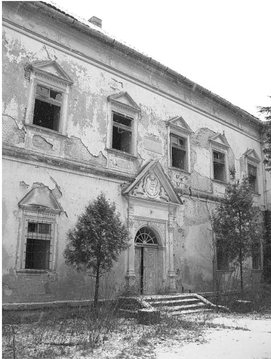
Fig. 10. Sânmiclăuș. The main entrance in the castle, edified by a splayed step pack. The short step parapets end by a pedestal. (photo: [www.monumenteromania.ro](http://www.monumenteromania.ro))
